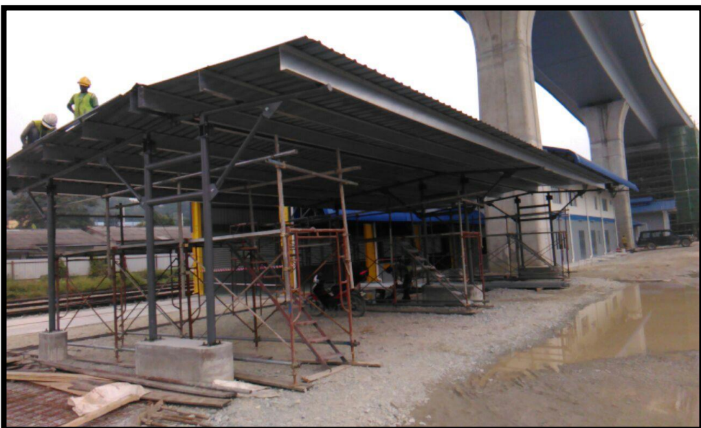
LUBRICANT STORE, SKID TANK & PARKING
