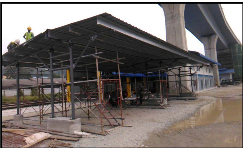
LUBRICANT STORE, SKID TANK & PARKING
