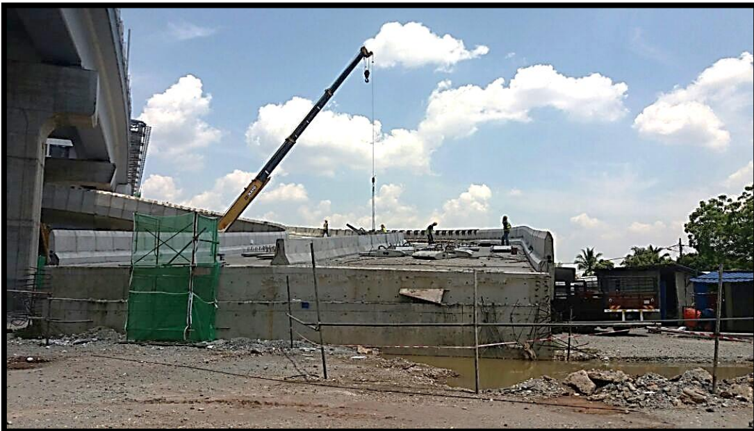
INSTALLA TION AND STITCHIN G OF NJB AND PARAPET WALLS
